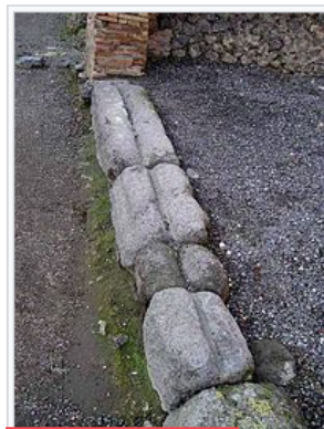
Roman sliding door tracks at Pompeii, Italy (1st century AD)
